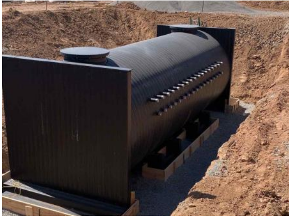
Geothermal vault is set in place (06/03/2022)
