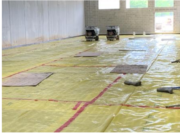
Wrestling room floor is prepped to receive concrete (06/28/2022)
