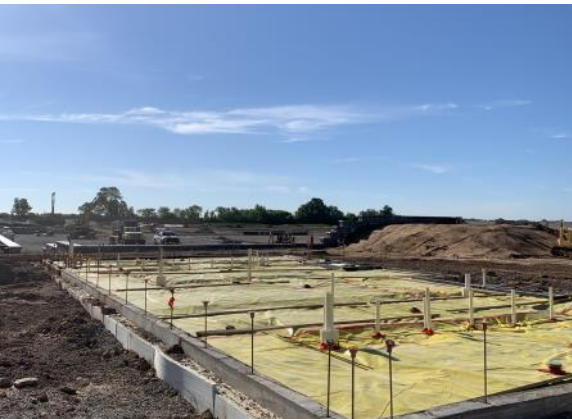
The North concession stand is prepped and ready for concrete (06/22/2022)
