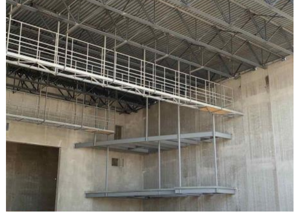
Catwalk steel in auditorium (06/03/2022)
